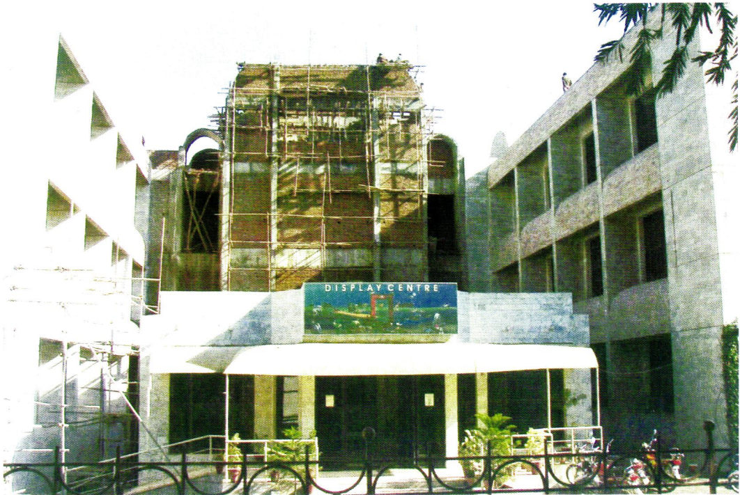
Under Construction Block II of PMNH
